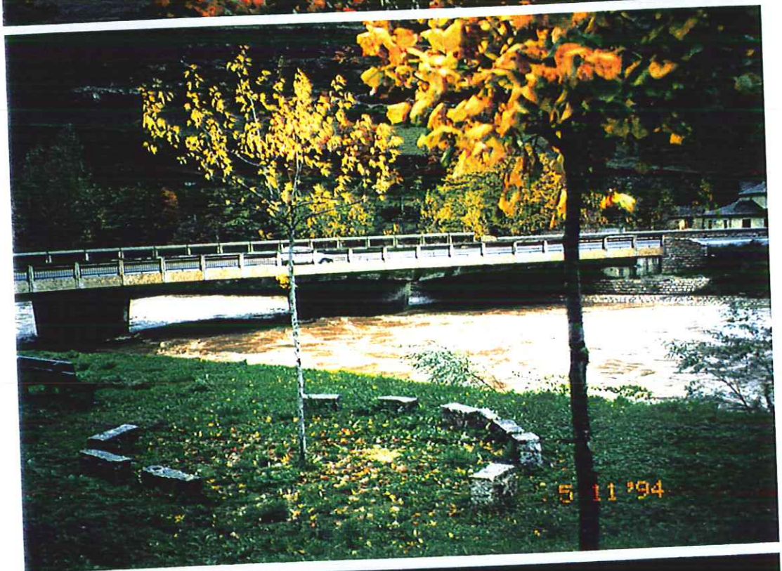
RN 88 PONT ST LAURENT
